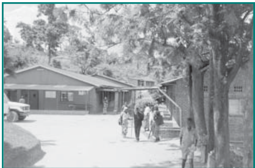
Kibogora Hospital, contains 198 beds, an Intensive Care Unit, lab, pharmacy, x-ray, and supportive facilities
