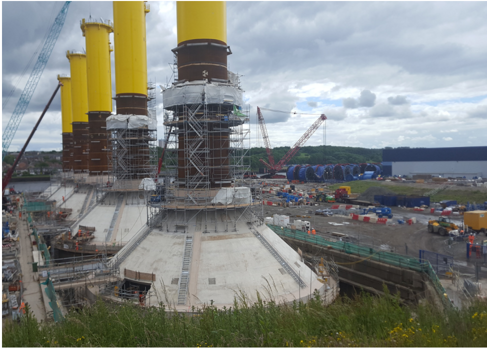
Figure 5 - Offshore wind turbine gravity foundations
