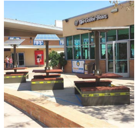
Figure 27. Outdoor seating with Solar Powered outlets.
