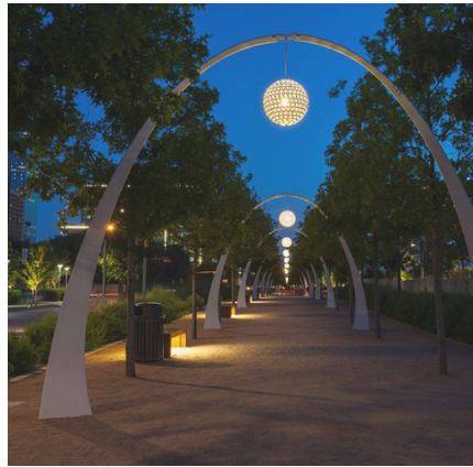
Figure 32. Pedestrian, park and bench lighting
