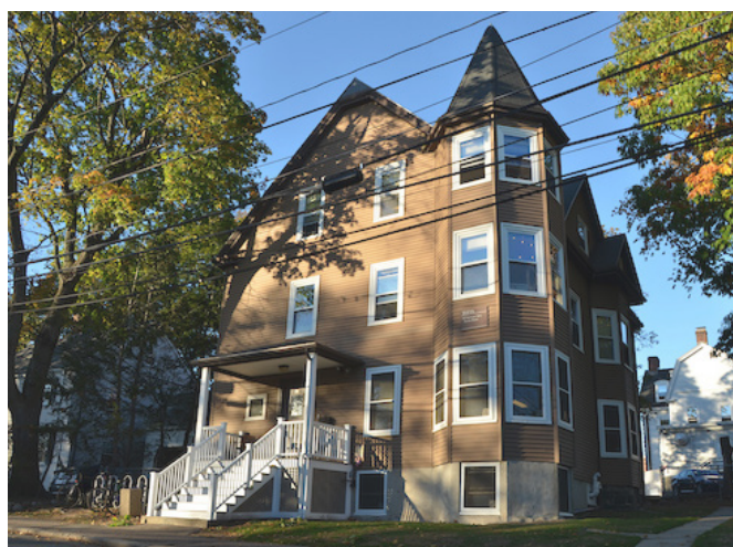
International House at Tufts University (Source: Tufts Daily)
