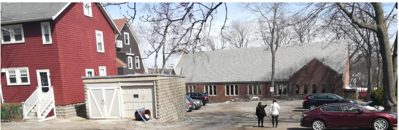
Figure 21. A small shed housing a garage also sits close to the Winthrop Street houses
