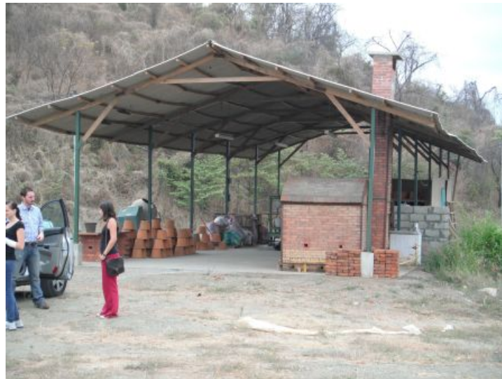
Figure 47: Hogar de Cristo Ceramic Filter Facility 2012 [98]
