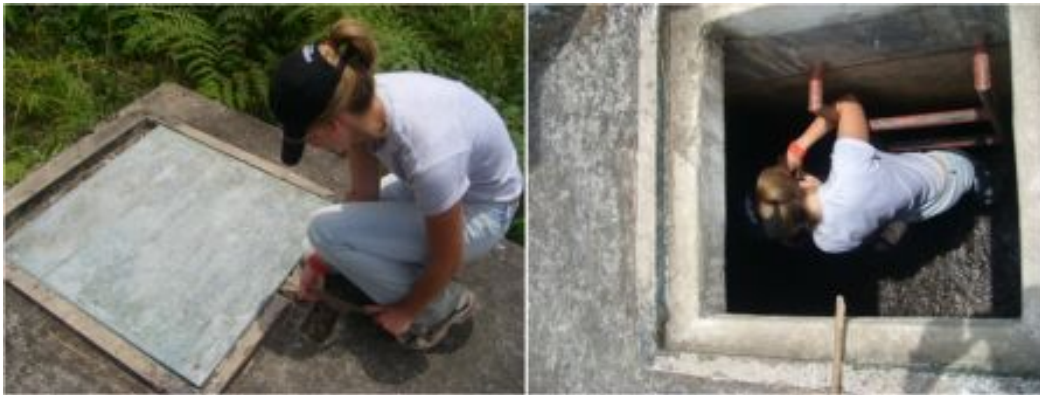
Figure 12: The distribution tank for El Cristal located after the slow sand filters. [55]
