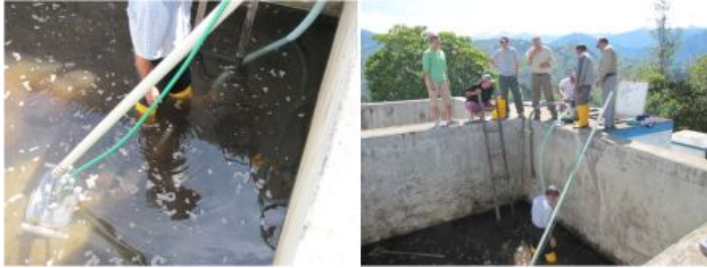
Figure 21: The siphon system developed by Tufts EWB [82]
