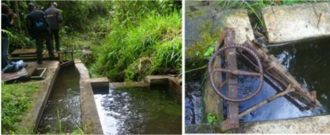
Figure 10: Capture tank for the El Cristal system. The Tufts EWB travel team noted that the tank was uncovered, but the entrance to the tank was a wire mesh in need of repair. [55]
