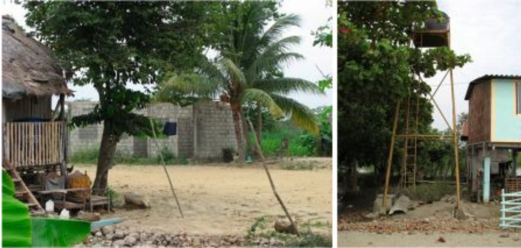
Figure 35: Semi-completed health clinic 2008 (left) and unused well and storage tank 2011 (right) [92]
