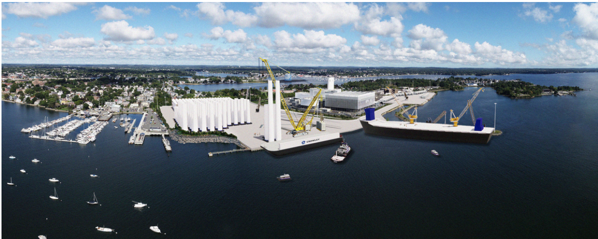
Image: Crowley Wind, Salem Offshore Wind Terminal
