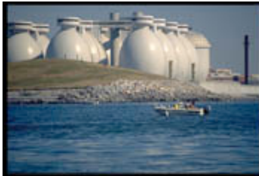
Municipal Waste Water Anaerobic Digesters at Deer Island in Boston Harbor.
